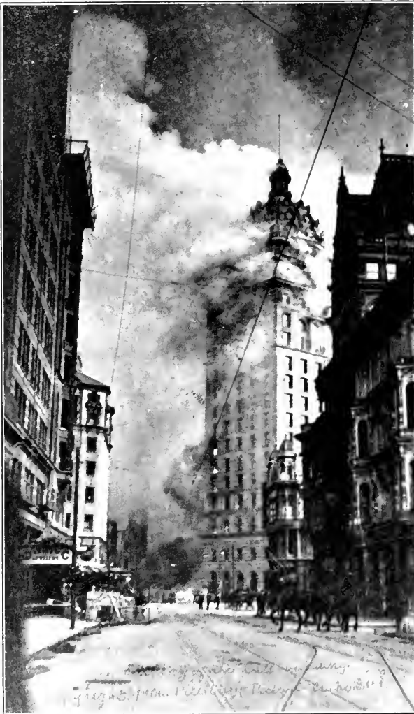
FIRE'S INGRESS via THE WINDOW ROUTE.
